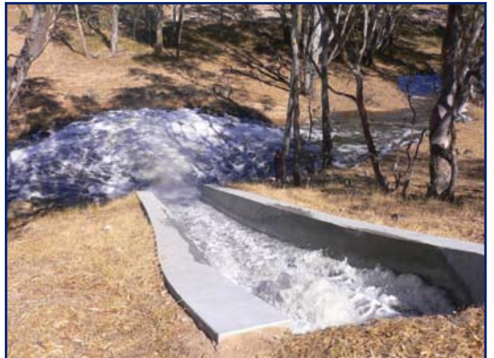
12-mile outlet during testing in March 2009. Releases were gradually increased up to a maximum rate of approximately 200 megalitres per day which is shown above.
